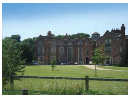
Danny House Hurstpierpoint
